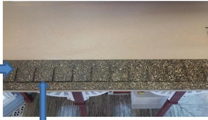
Lower shingle divider line is align center to top shingle.
